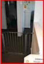
21430 Dead stop on the stairs
