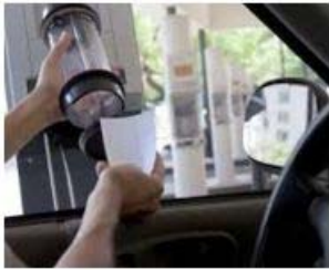
Suction canister at the drive-in teller (drive-in bank)
